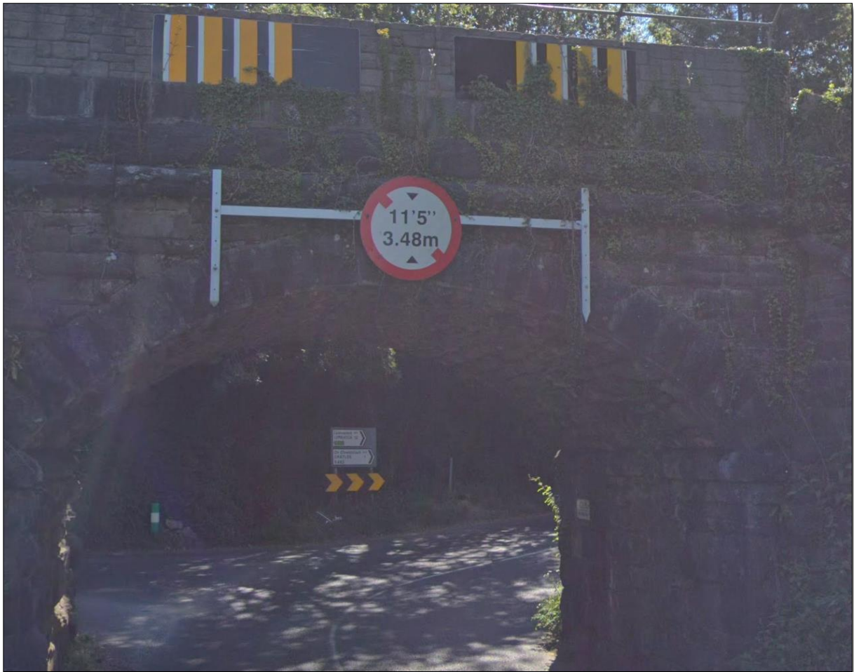
Figure 5 Bridge on approach to Sixmilebridge
